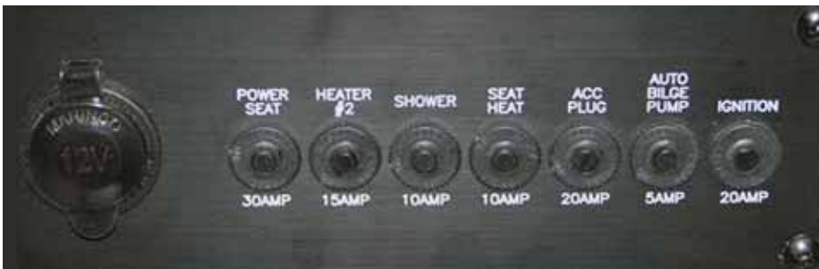
Figure 2-13. Circuit Breaker Panels
