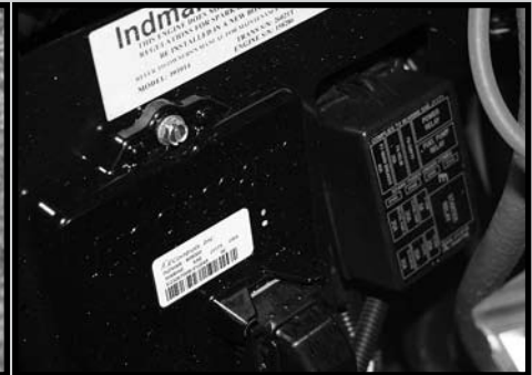
Fuse Panel - Back of Engine
