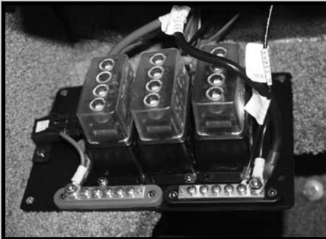
Fuse Panel - Under Dash
